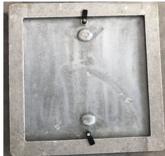
Manhole Covers with Anti-Corrosive Locks
