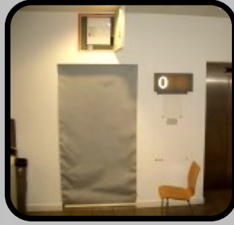
...to cover elevators openings
