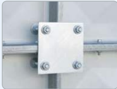
3. External reinforcement (Lower piece—HDG)
