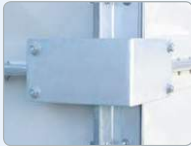
2. External reinforcement (Corner piece—HDG)
