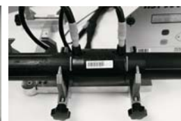
Phase 7 welding and cooling
