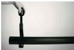
Phase 1 cutting of the pipe
