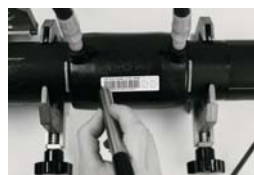
Phase 6 setting up of welding parameters with bar code reader
